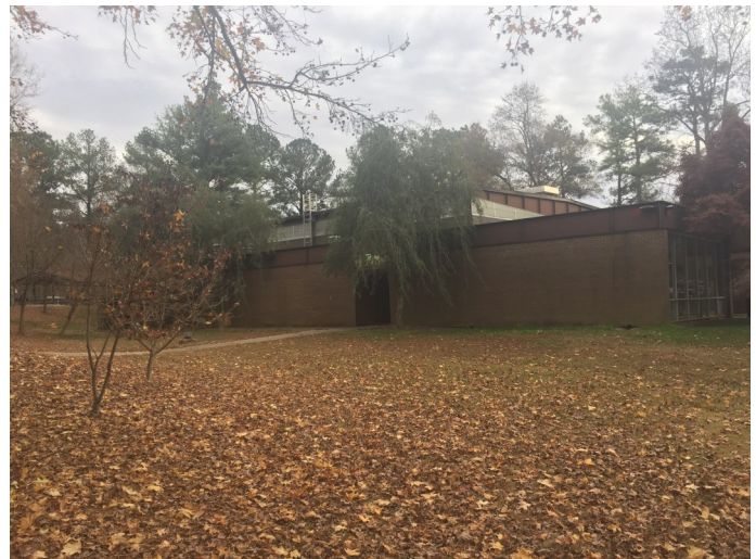
Biltmore Hills Community Center Side View
