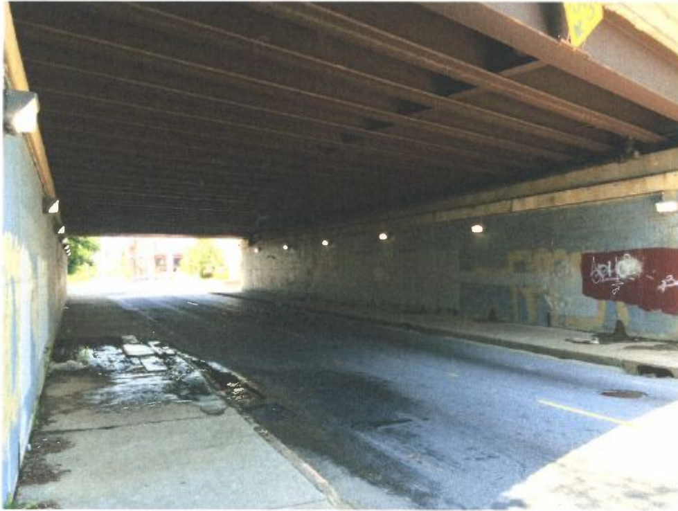
Interior Underpass Existing Condition
