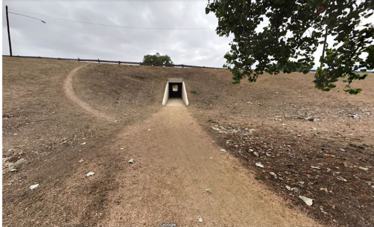
Existing Pleasant Valley pedestrian underpass – Looking east
