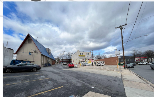
#3. View from Ennalls Ave
