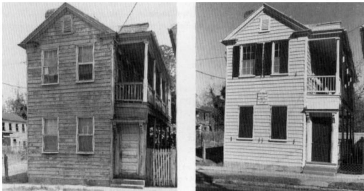
*Maximizing retention of historic materials and features is the primary goal of Preservation as demonstrated here in these “before” and “after” photographs. Aside from some minor repairs and limited replacement of deteriorated material, work on this house consisted primarily of repainting the wood exterior. Photos: Historic Charleston Foundation.*
