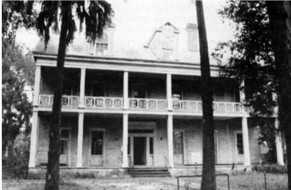
*The Bronson-Mulholland House in Palatka, Florida, ca. 1845, is shown (a) before and (b) after the treatment, Restoration. Over the years the east (far right) side of the veranda had been filled in as a sixth bay. During the restoration, this later infill was removed and the east veranda, together with its flooring, stairs, and foundation, restored. Photo: City of Palatka, Community Development Department.*
