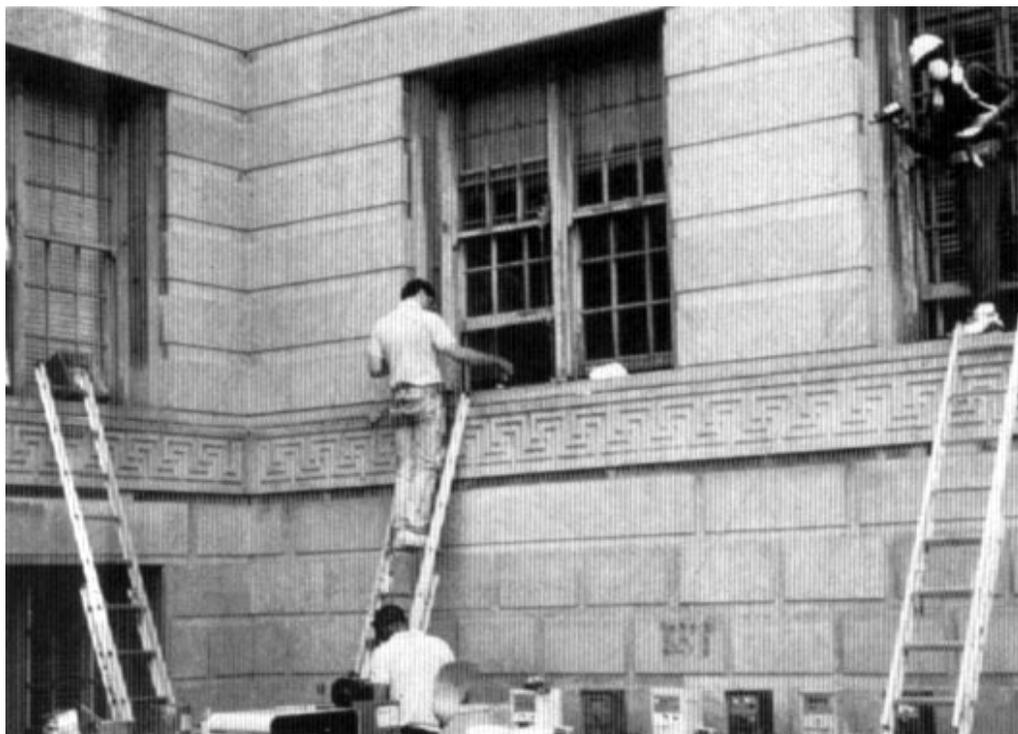
*Preserving a building's historic windows generally involves scraping, sanding, and re-painting. While some repair work will most likely be undertaken within the scope of work on this institutional building, replacement of the window units is usually not an appropriate Preservation treatment. Photo: Chuck Fisher.*
