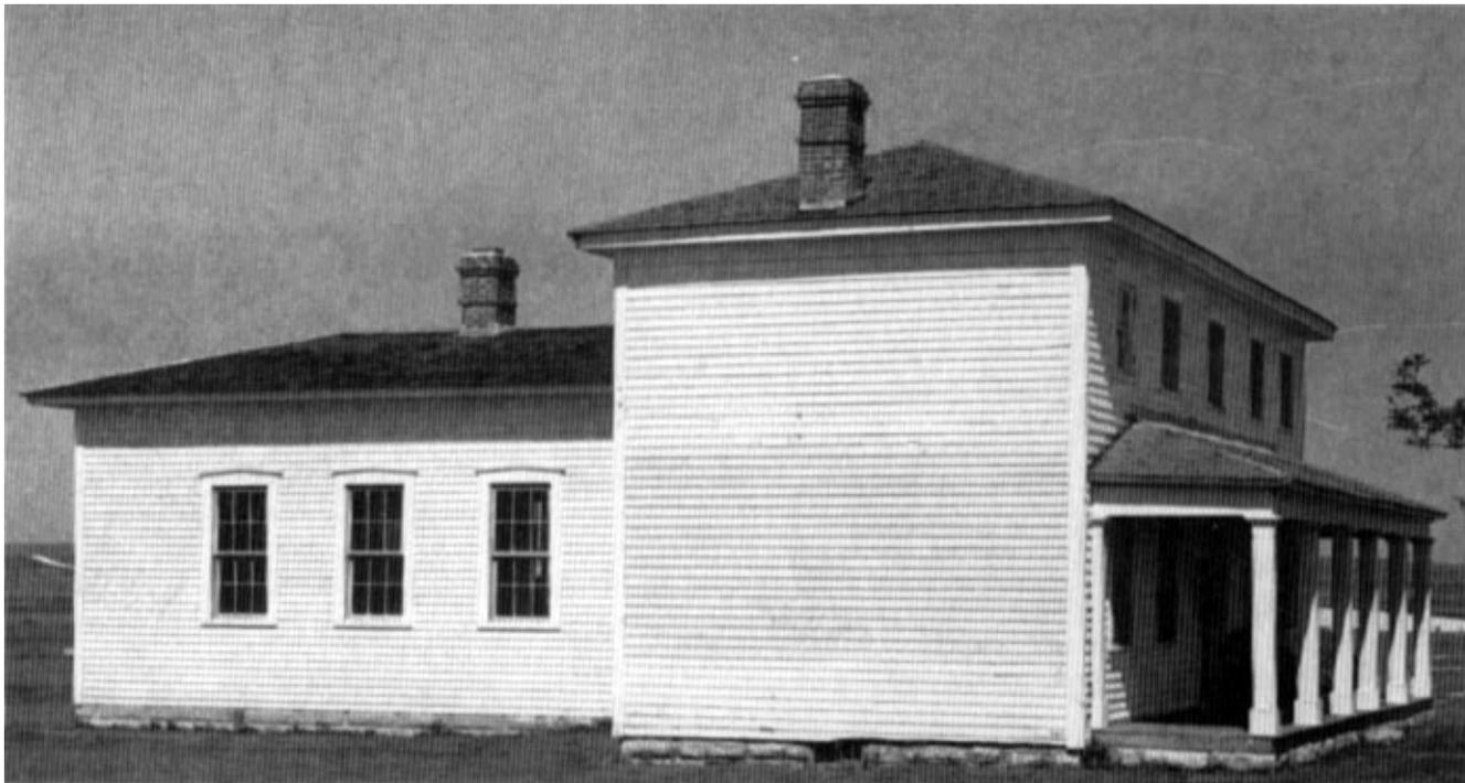
*In a project at Fort Hays, Kansas, the wood frame officers' quarters were restored to the late 1860s—their period of significance. This included replacing a missing kitchen ell, chimneys, porch columns, and cornice, and closing a later window opening in the main block. The building and others in the museum complex is used to interpret frontier history.*
